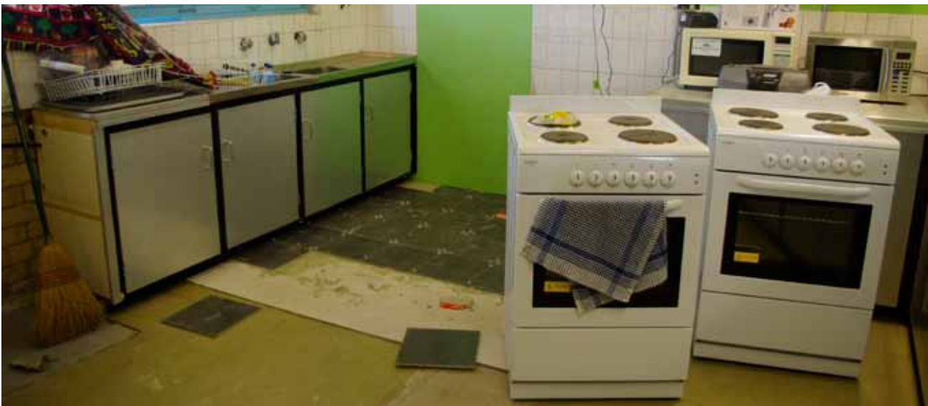
Figure 3.7 Kitchen construction in progress
