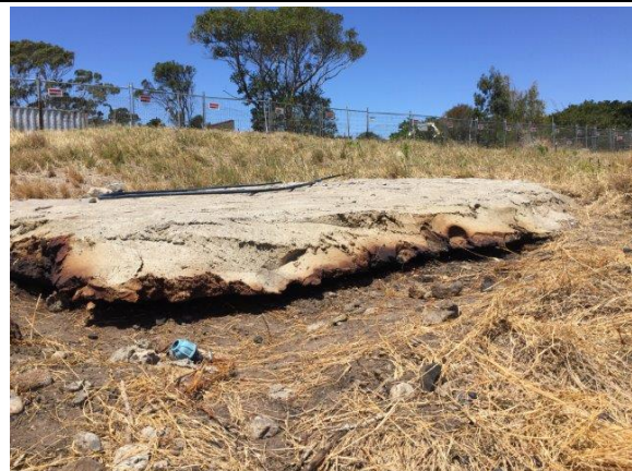
Photo 2. Initial Site Assessment – 31 st October 2017 – Area of Concrete Pad
