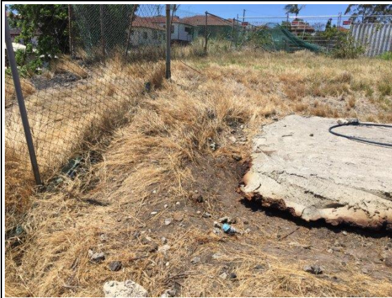
Photo 1. Initial Site Assessment – 31 st October 2017 – Area of Concrete Pad and internal fence
