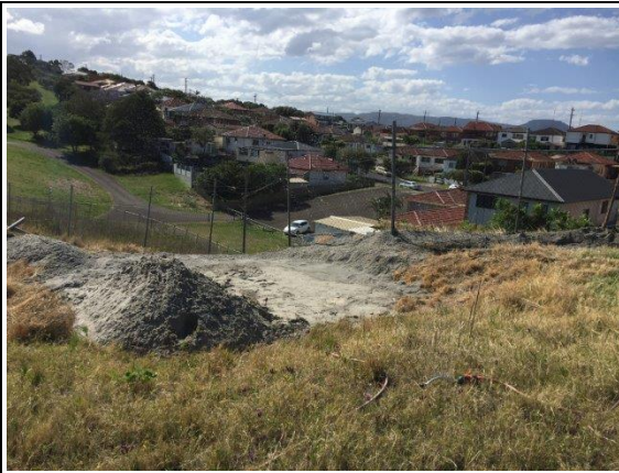
Photo 5. Initial Site Assessment - 31 st October 2017 - Area of Concrete Pad and internal fence covered with wet sand
