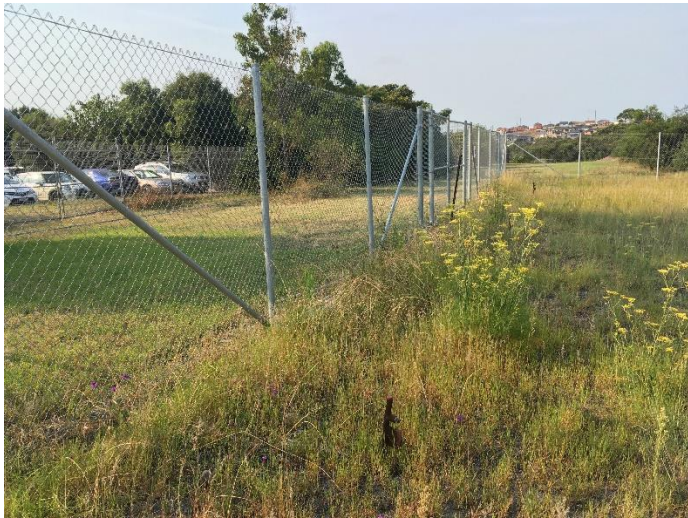
Picture 1 – Exclusion zone fencing surrounding north-western hotspot area
