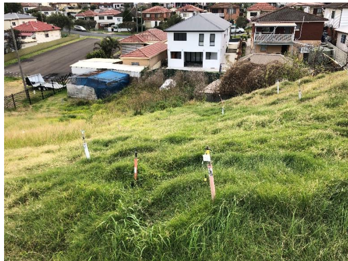
Picture 3 – Slope within north-western hotspot area
