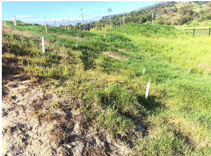
Picture 3 – Slope within north-western hotspot area
