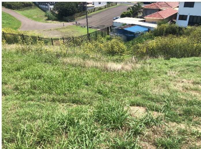
Picture 3 – Slope within north-western hotspot area
