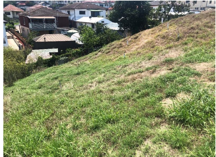
Picture 2 – Slope within north-western hotspot area
