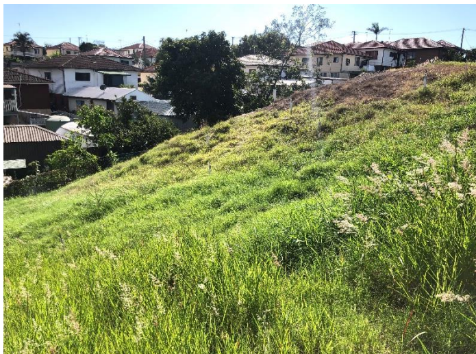
Picture 3 – Slope within north-western hotspot area
