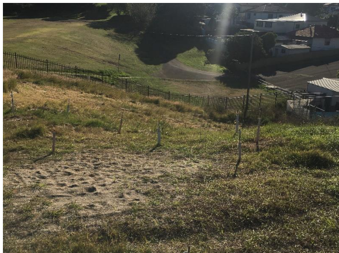
Picture 3 – Slope within north-western hotspot area
