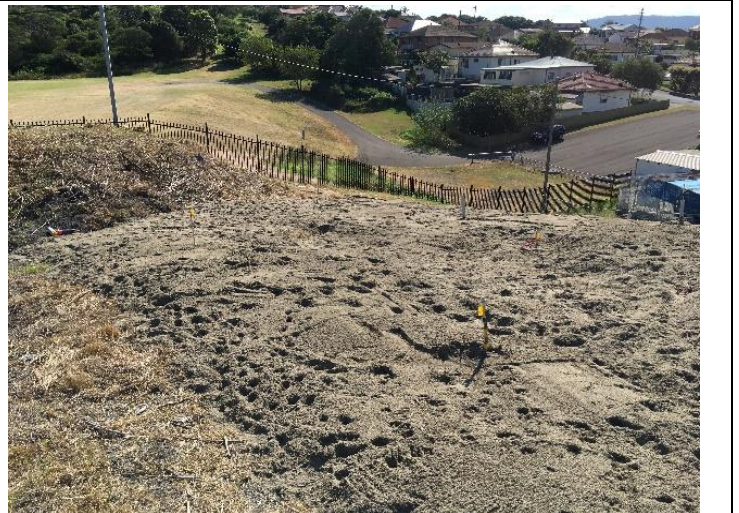
Photo 10. Placement of Sand across area of concern - April 2018
