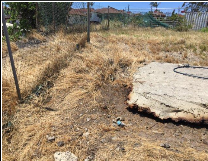
Photo 1. Initial Site Assessment - 31 st October 2017 - Area of Concrete Pad
