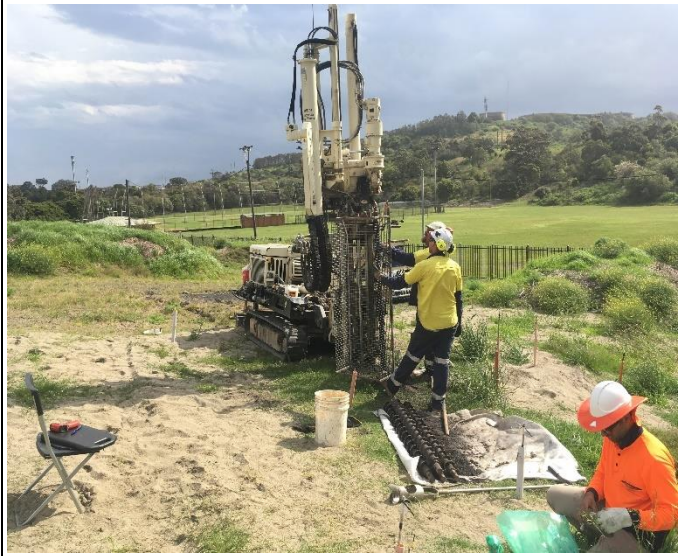
Photo 13. Geotechnical investigation and Installation of Subsurface Thermocouples – October 2018
