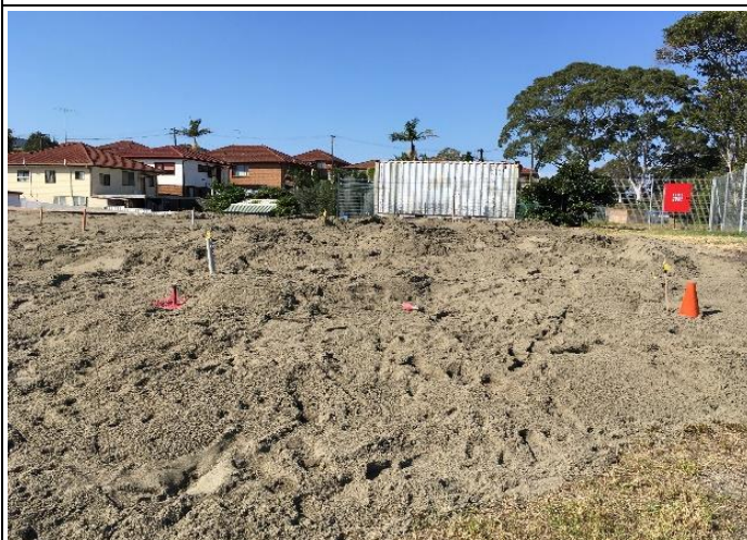
Photo 11. Placement of Sand across area of concern - April 2018
