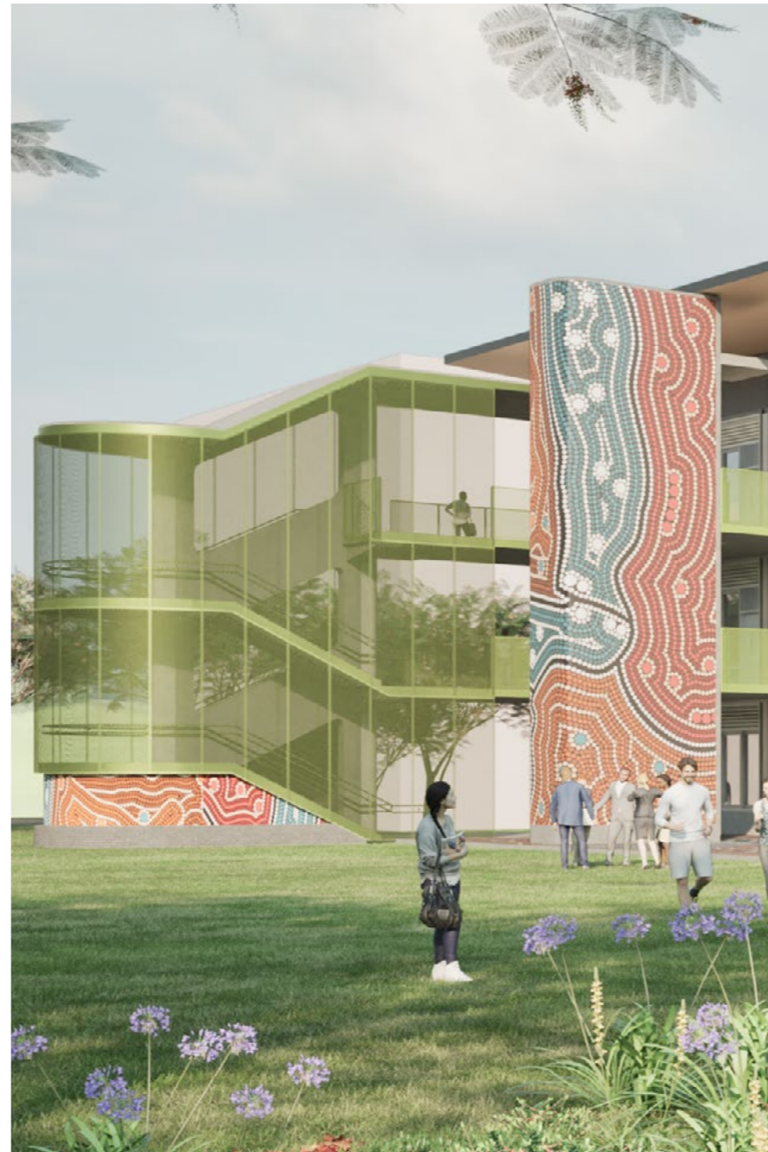
Concrete painted with artwork
