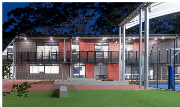
Classrooms and courts, Cherrybrook Technology High School
